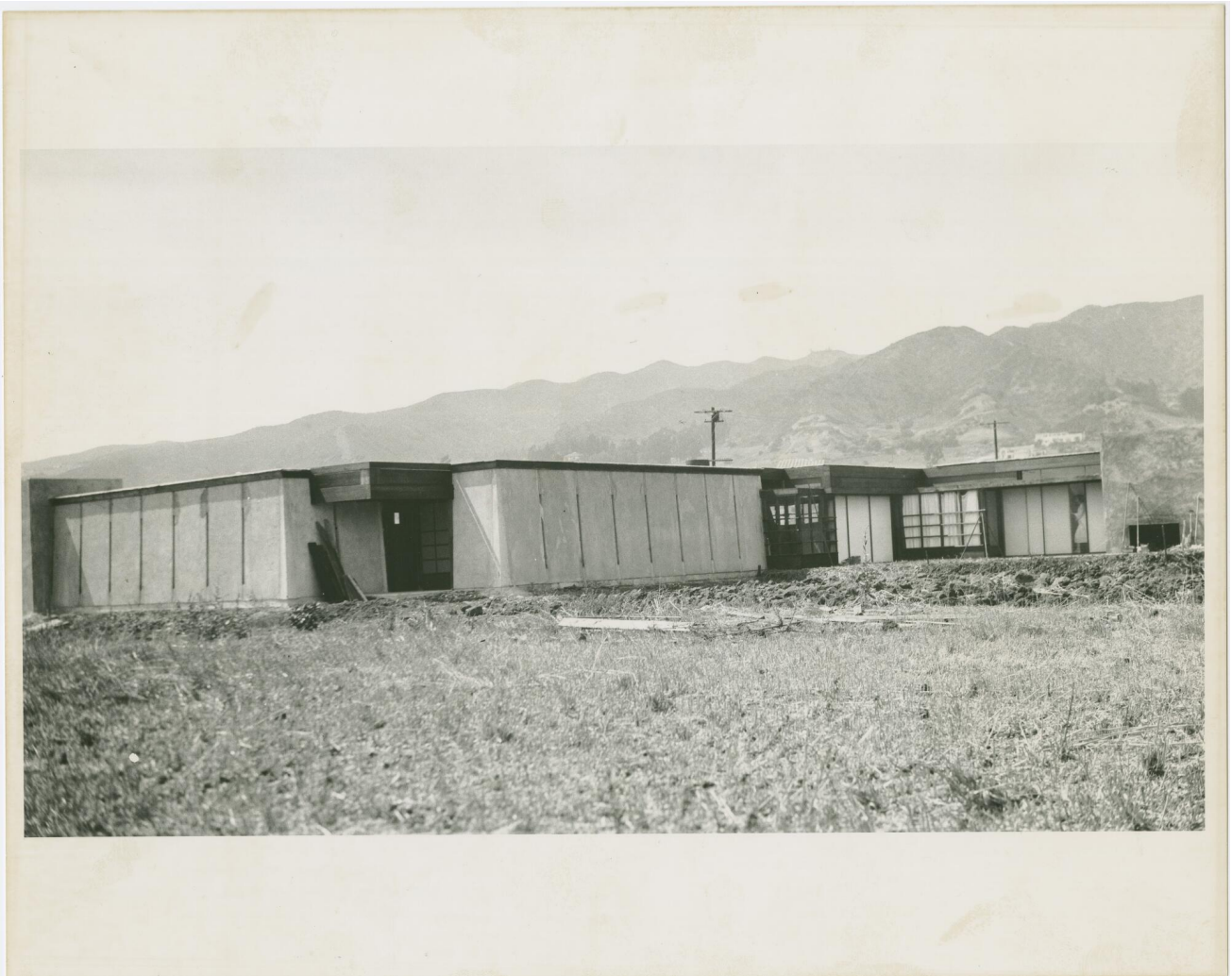
A view of the nearly finished Schindler House in the 1920s in what is now West Hollywood.
